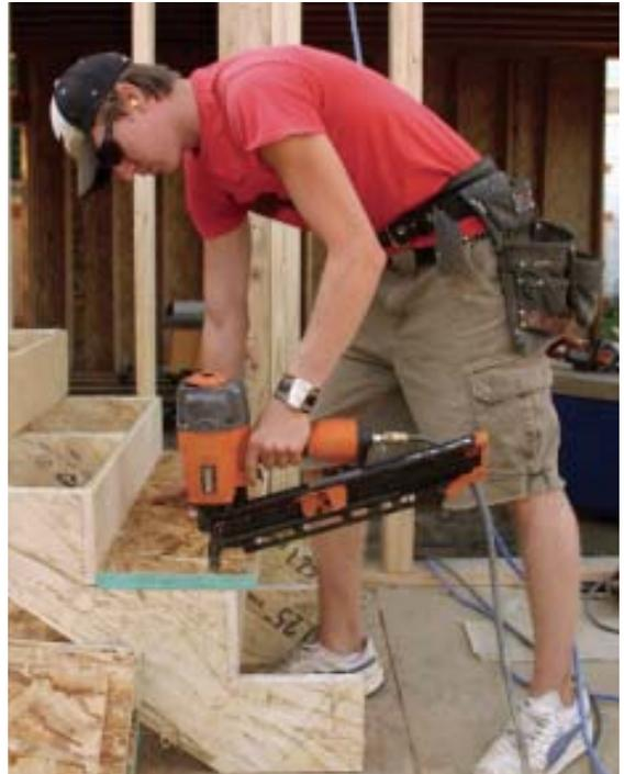
Other features include an adjustable exhaust cap, tool-free depth of drive, and a muffler to dampen sound. I appreciate these features, too — but nowadays just about every tool has them so they aren't worth getting excited about.
